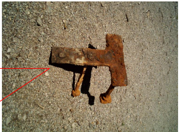
Supporting brackets from a picture of Lock Seven on the Seven Locks Flight at Tockenham. Taken in 1970. The example above from Pewsham Top Lock is very close in comparison.
