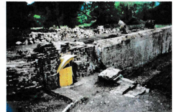
Restoration of Bottom Lock at Pewsham
